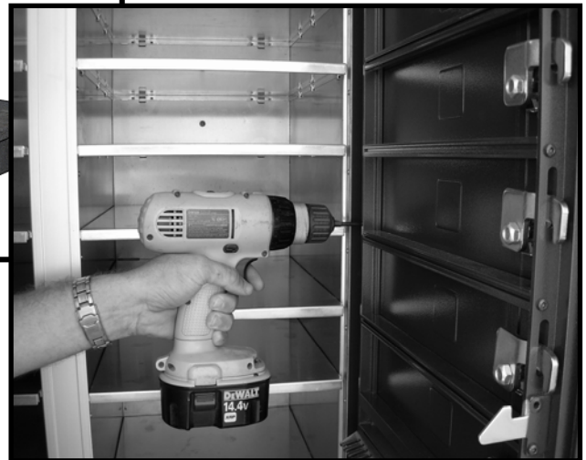
Figure 2 – removing mounting screws
