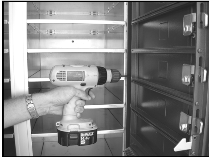
Figure 19 – Securing versatile™ module to DEPOT™ stand
